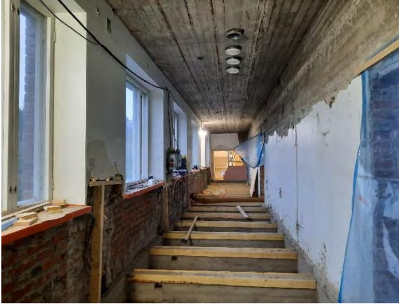
Härmälä School renovation site, intermediate floor filling suction/cleaning work
