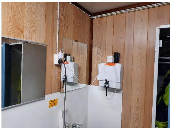
Construction site shed, surveyors measuring
