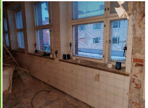
Härmälä School Renovation construction site, surveyors taking measurements
