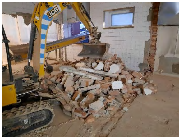
Härmälä School renovation , concrete/brick debris cleanup
