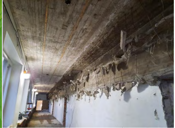
Härmälä School renovation construction site, concrete beam demolition work
